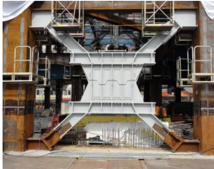
An Fe-Mn-Si based vibration damper unit. JP Tower Nagoya, Japan
